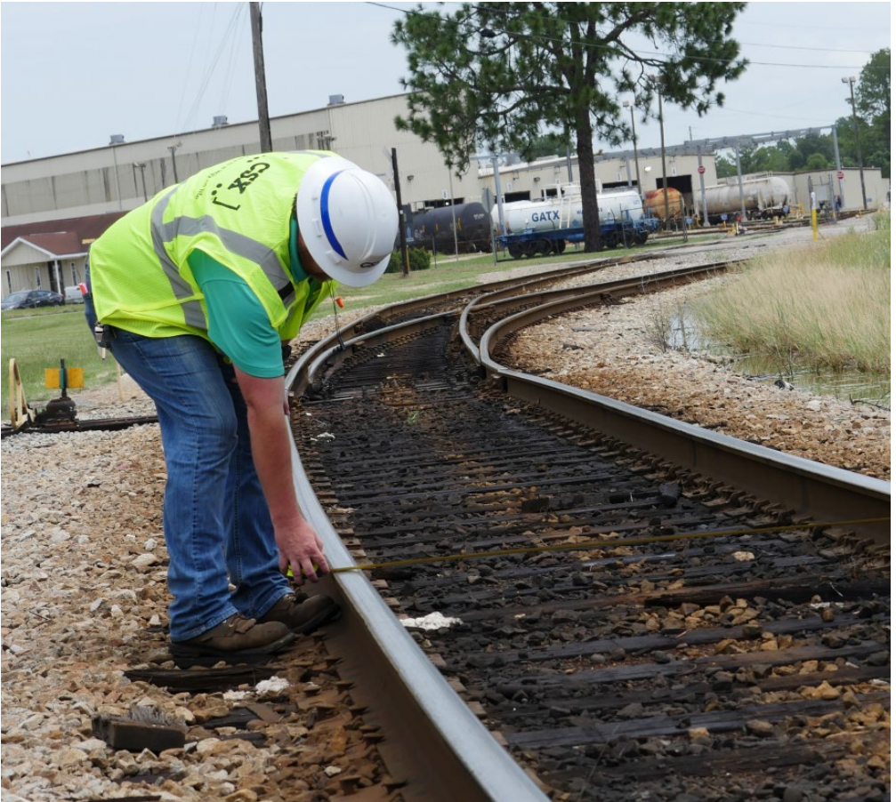
Inspect tracks, switches and signals
