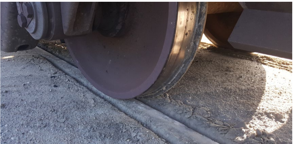
An example of muddy conditions that can contribute to degradation of track
